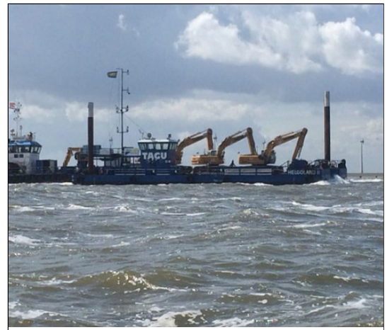
October 2014 to June 2015 (Engineering and Construction Phase)
