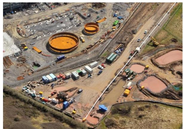
Pipe String entering the Bore at the Power Station Drill Site
