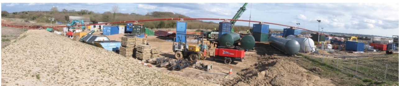
Pipe String Overbend at Lepe Drill Site
